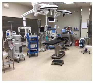
A poured-in-place urethane mortar system provides this orthopedic surgical suite with weldless, long-lasting, stain-resistant floors.
