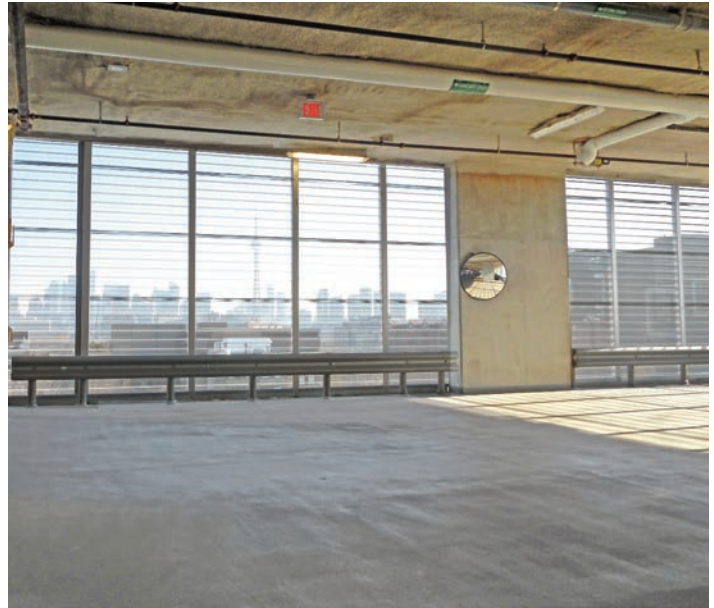
New construction before installation of Stondeck XD2 for superior protection.
