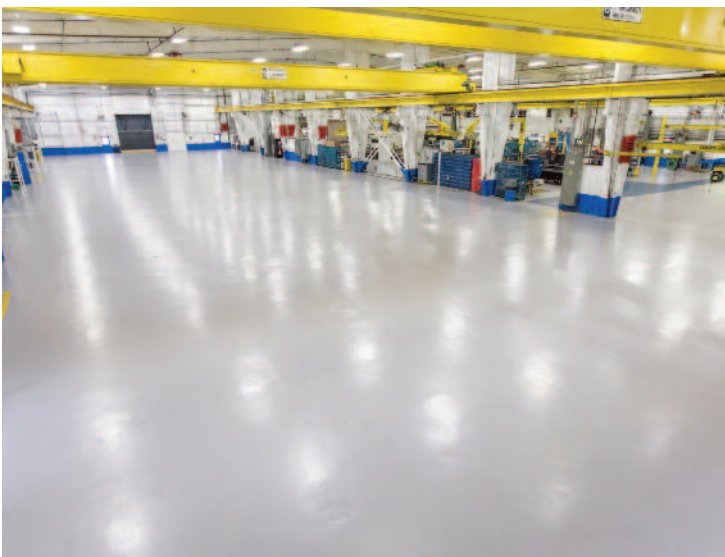
Stonclad GS replaced severely worn, oil-soaked concrete
