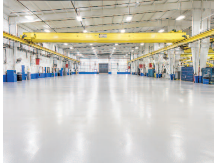
Baker Hughes machine shop became a showcase for customers after the installation of Stonclad GS
